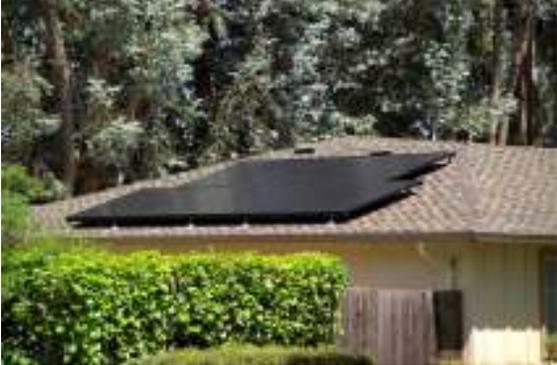
(Non compliant street side roofs with exposed and metallic mounting hardware and lack of symmetry in application of equipment.)
